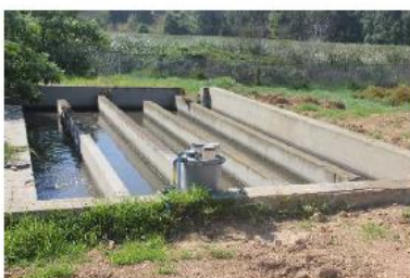
Chlorine contact channel
