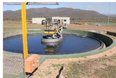
Secondary Settling Tank
