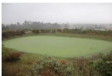
Anaerobic Pond No. 1
