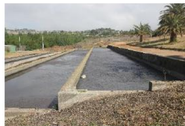
Sludge drying beds
