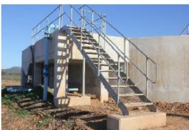
Raised Inlet structure
