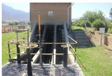
Archimedes screw pumps
